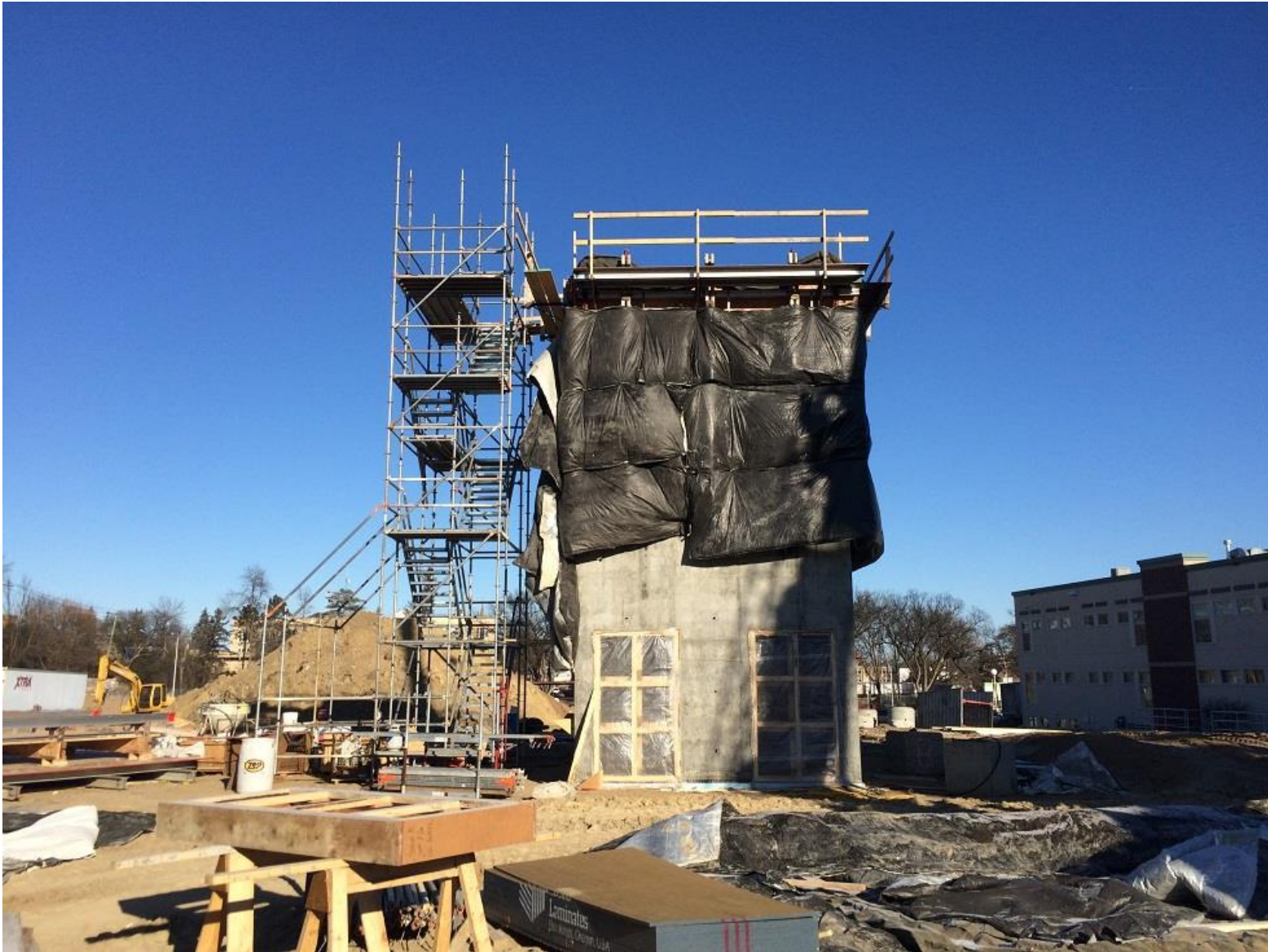
2 nd level of the elevator core walls poured.
