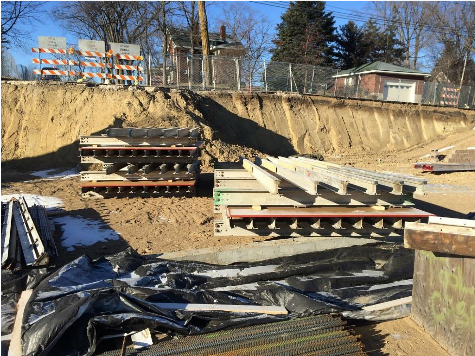
Forms delivered and being prepped for Stair A core walls.
