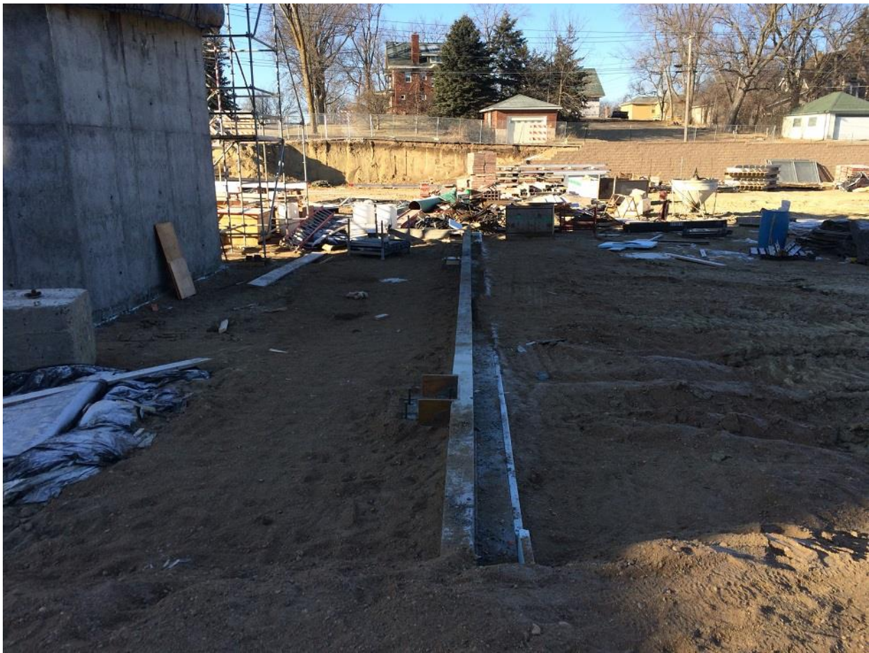
Foundation footings and grade beams completed .
