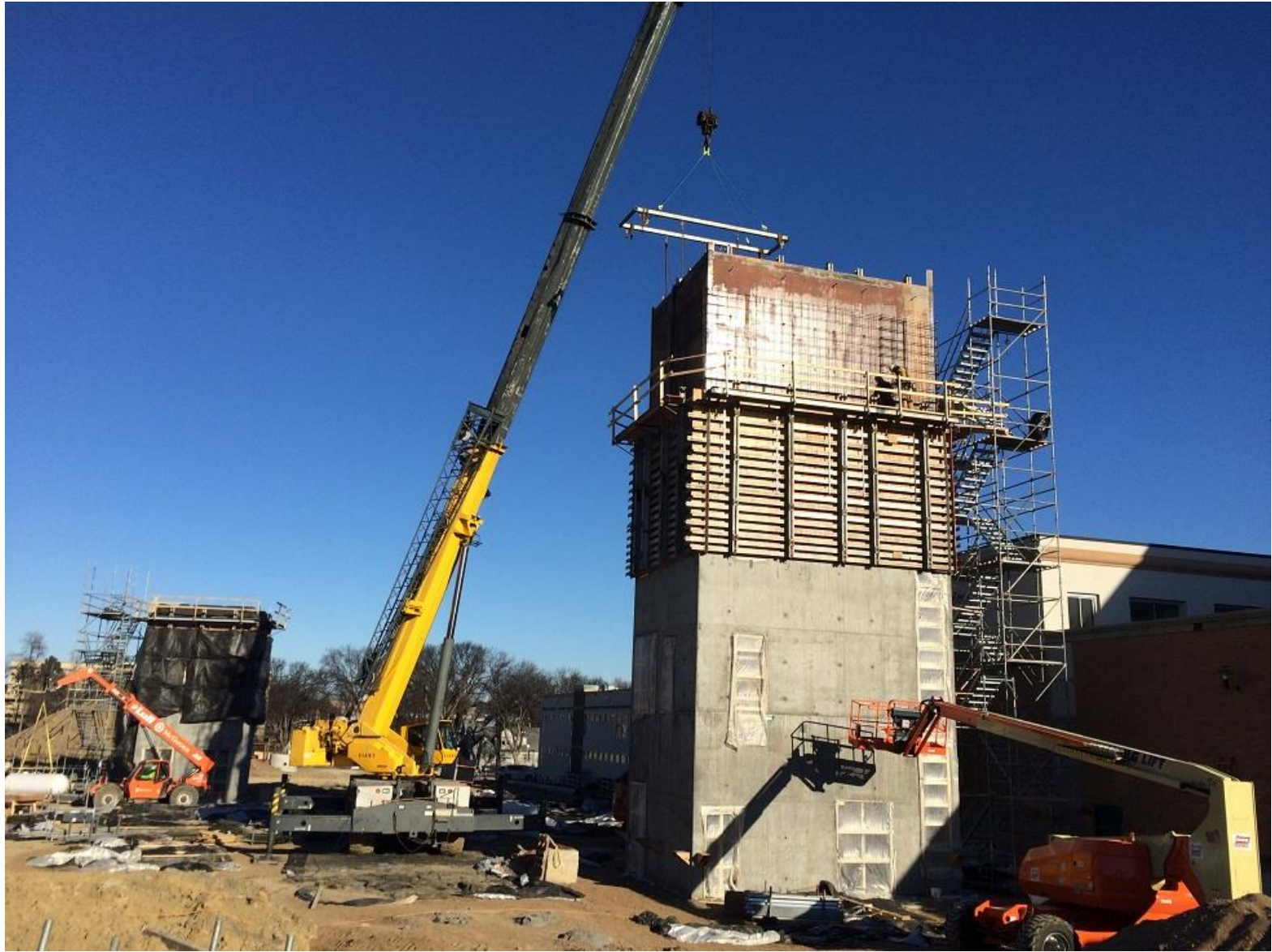
Stair B 3 rd level poured and beginning to form 4 th and final level.
